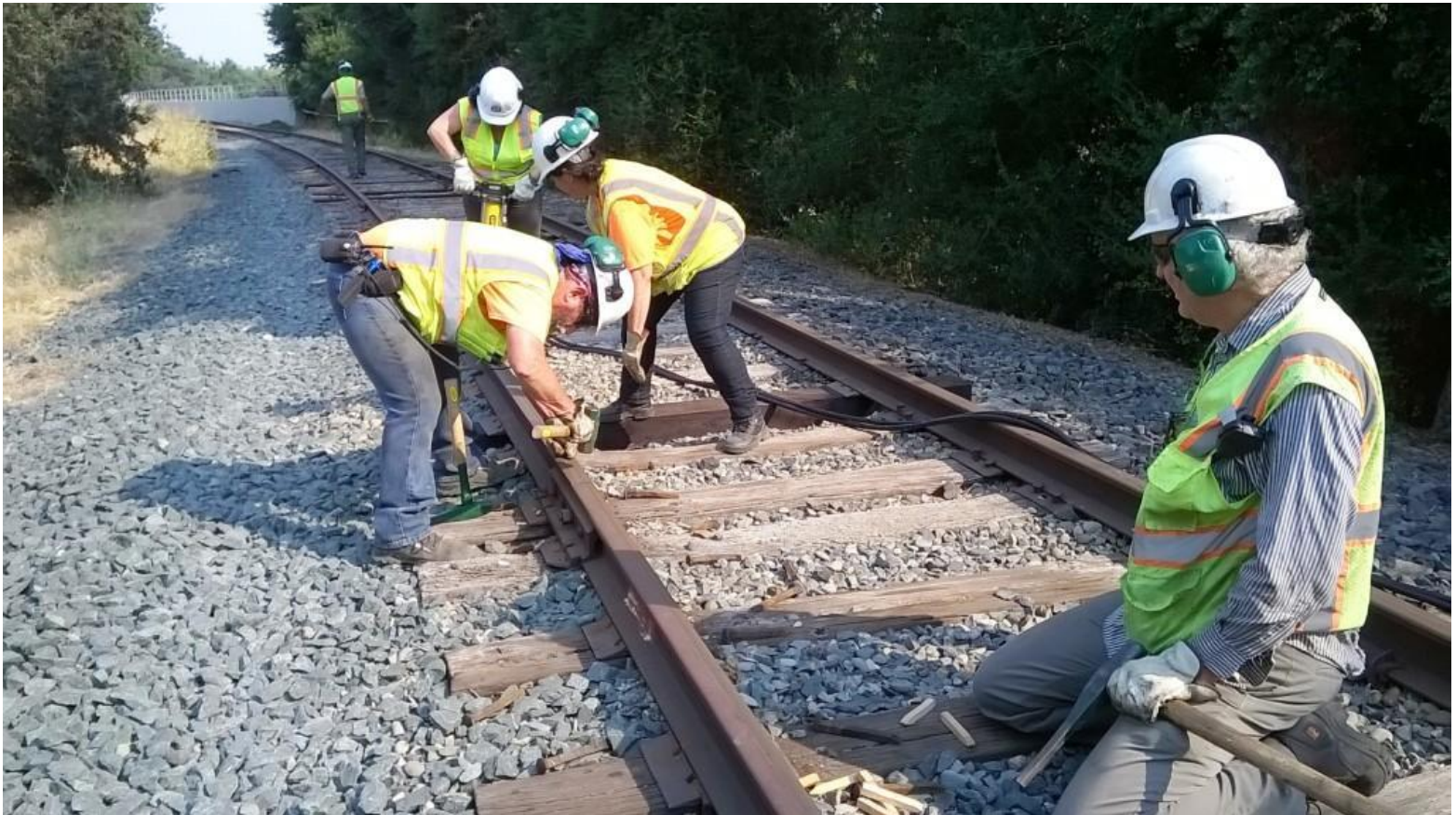
Now mechanized, Team Gauging make huge progress. Mary pulls spikes with the hydraulic spike puller and Pam, Joe, and Steve plug spike holes
