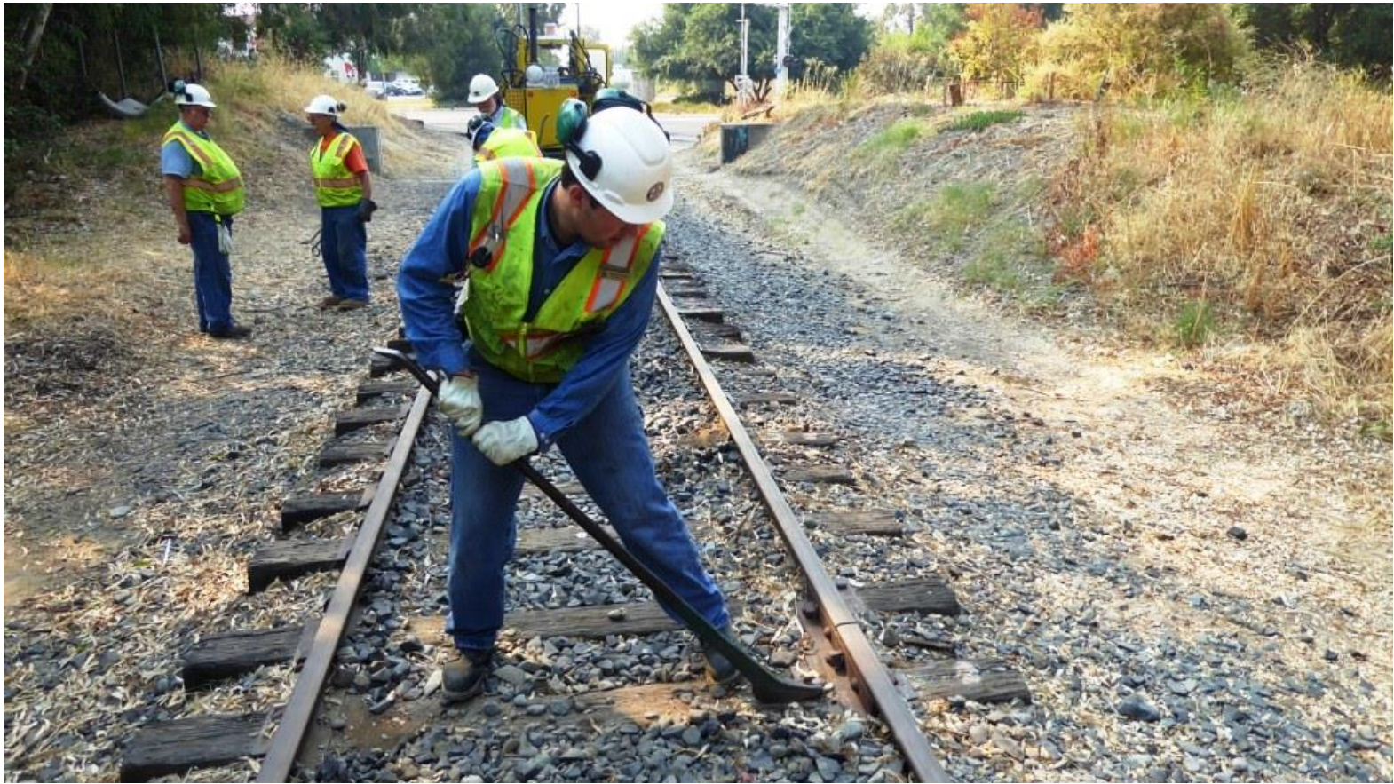
Weston, on Team Tie-shear, pulls spikes
