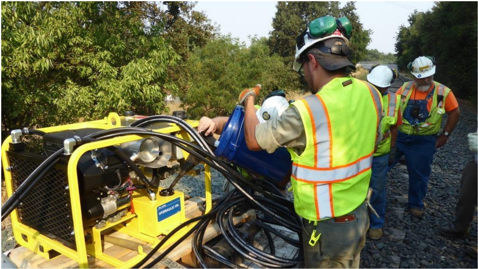
Kyle and Chris add hydraulic fluid to the new hydraulic power unit – our first brand new piece of equipment in memory
