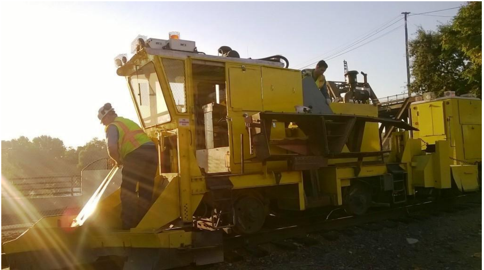
Chris and Weston open up the ballast regulator to use it to trigger the interlocking signals for crossing the UP Main
