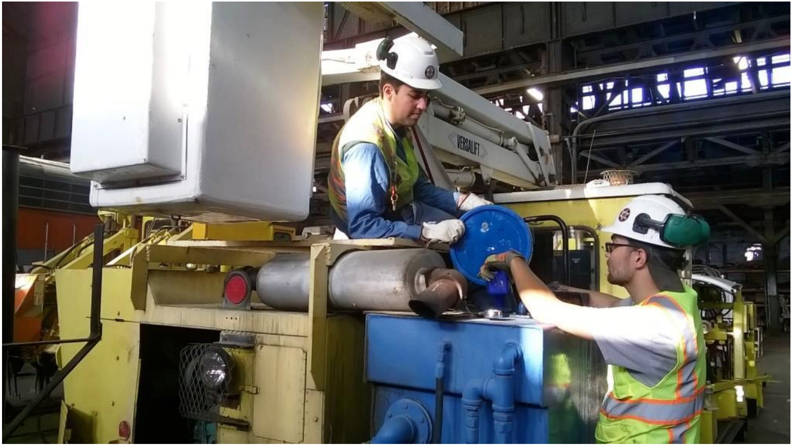
Weston and Kyle add hydraulic fluid to the man-lift's hydraulic tank
