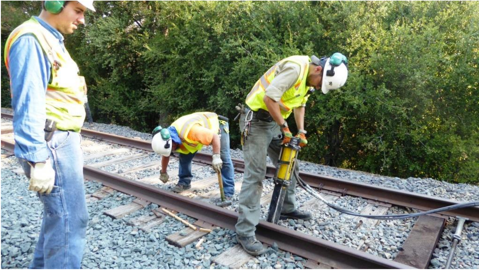
Now Kyle tests out the hydraulic spike-puller as Joe plugs old spike-holes with tie-plugs.
