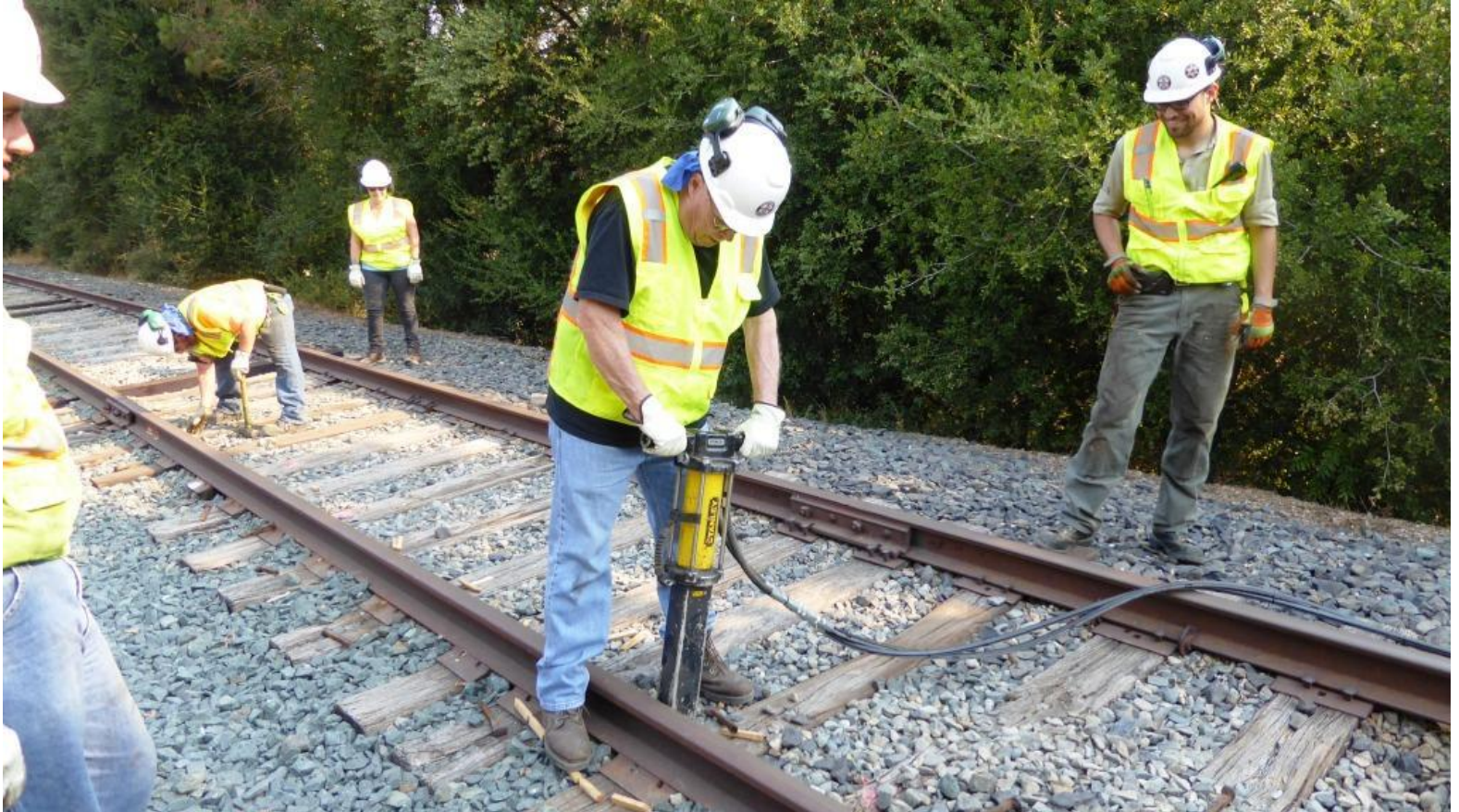
Bill's turn at the hydraulic spike-puller
