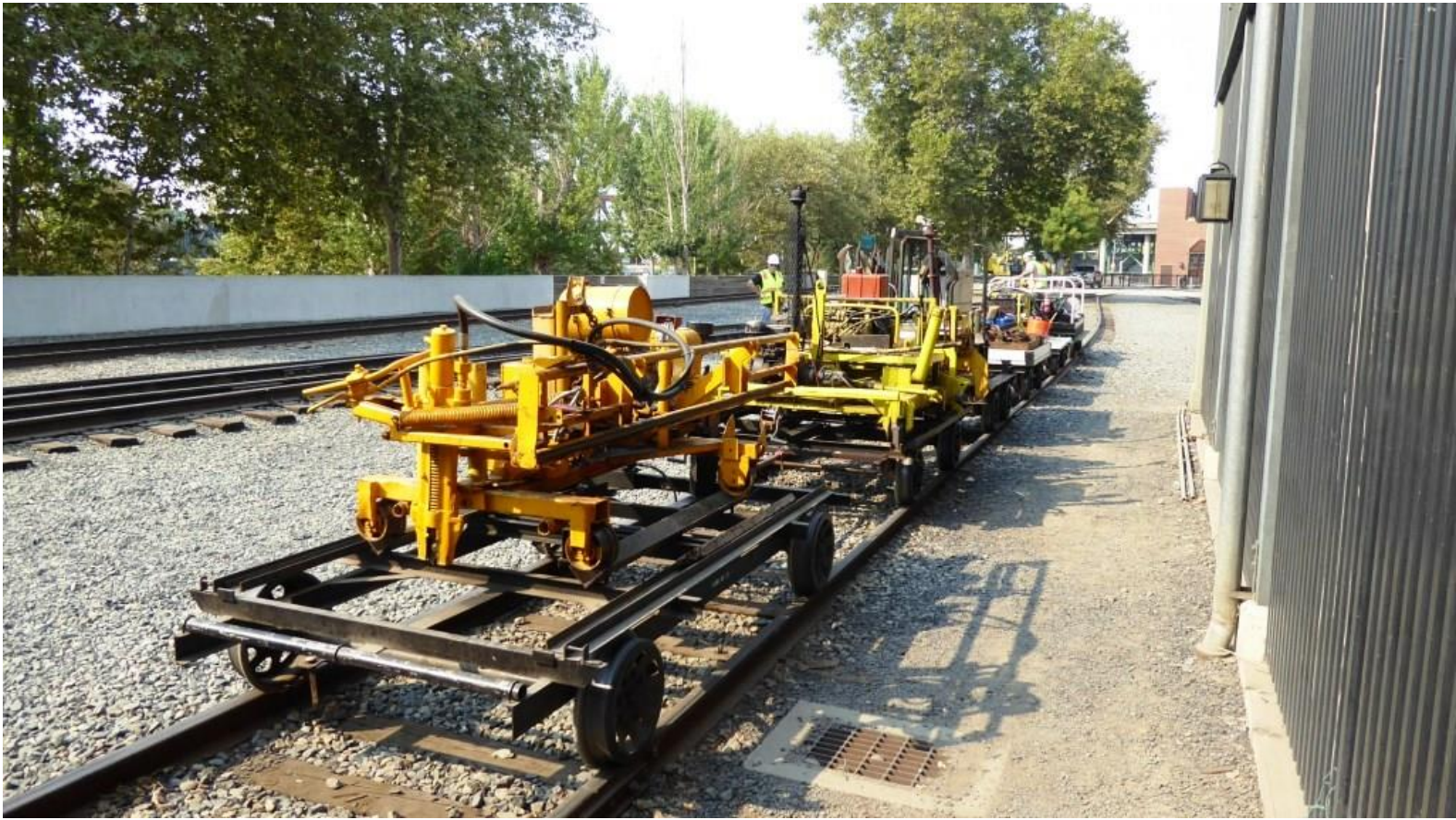
In Old Sac., Steve skillfully shoves the equipment into the container
