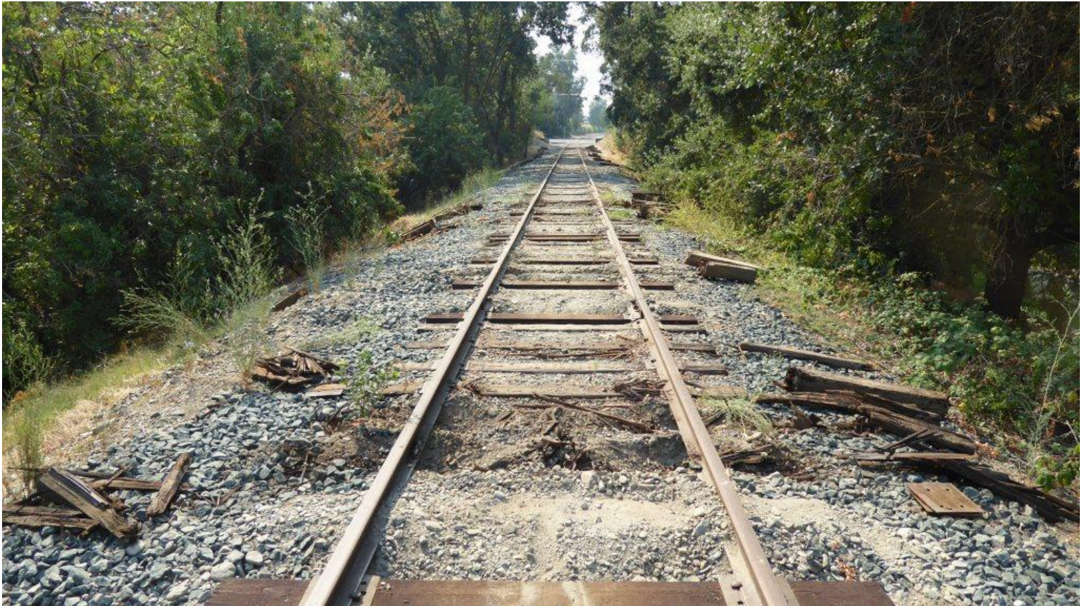
Clear evidence that the tie-shear has been on-site...
