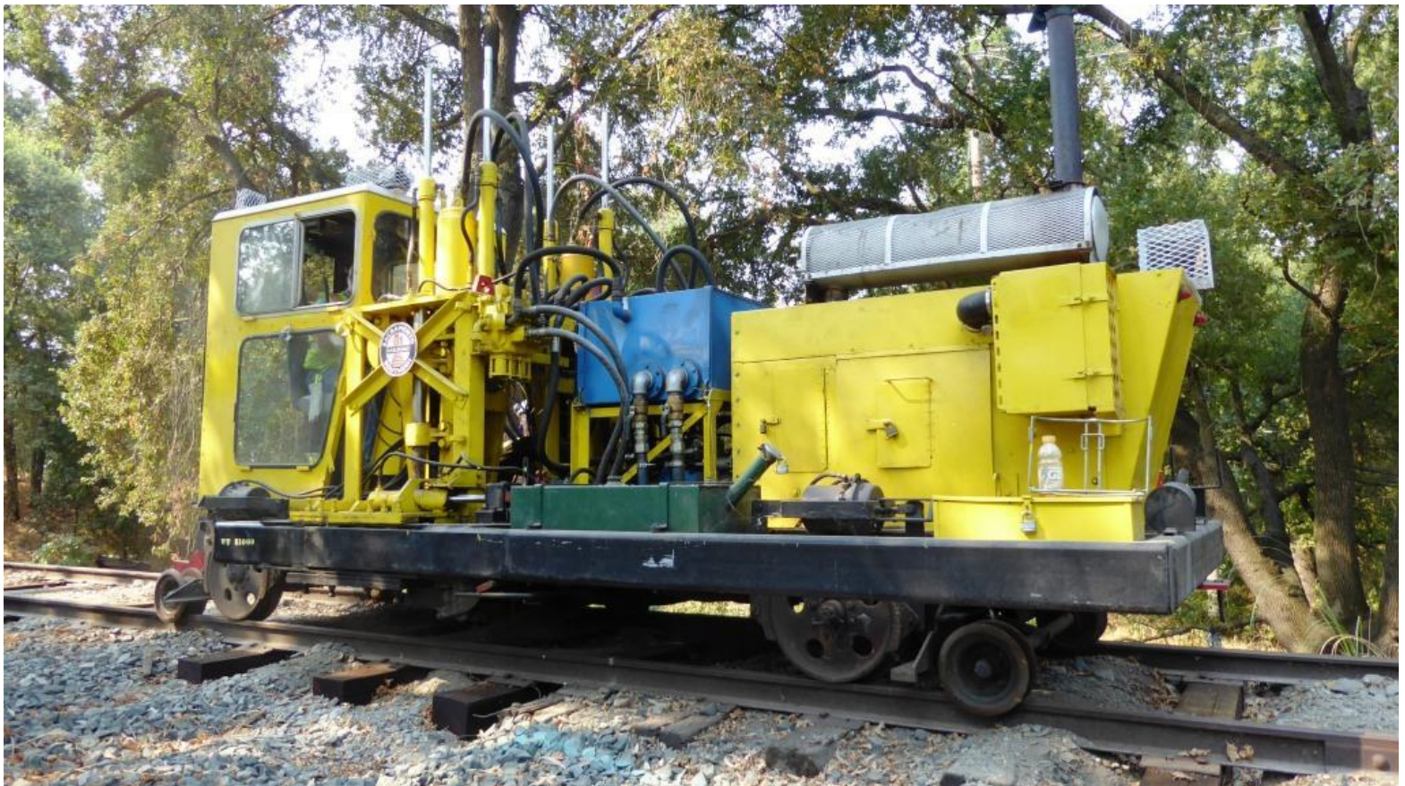
Chris brings in the tie-shear, and slices the ties into thirds, then kicks the pieces out the sides. This machine is awesome!
