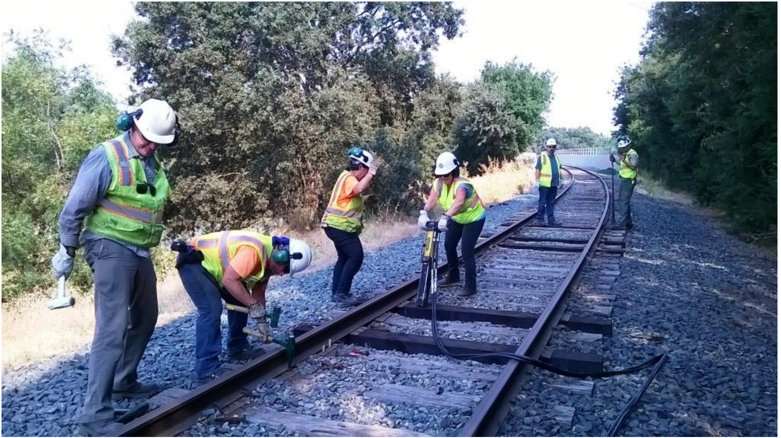
With the spike-pulling and driving now mechanized, the gauging operation went lickety-split
