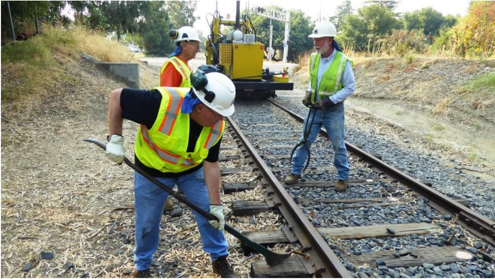
Bill, with Team Tie-shear, starts by pulling spikes...
